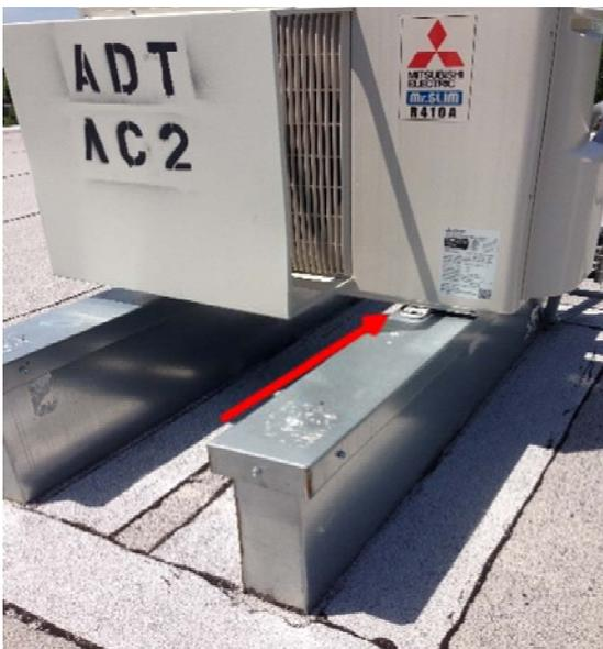
*Split HVAC unit not secured to its curb*
