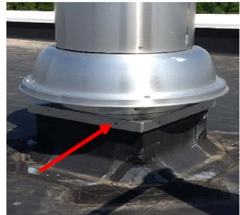
*Exhaust fan with no base fasteners*
