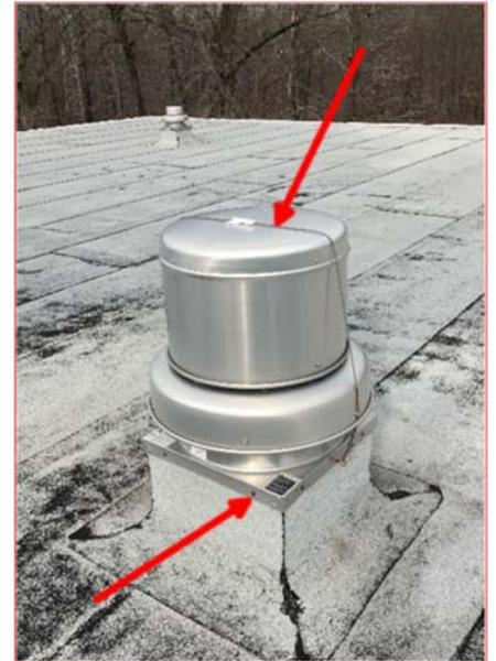
*Well secured curb mounted exhaust fan; use two straps in high wind zones*
