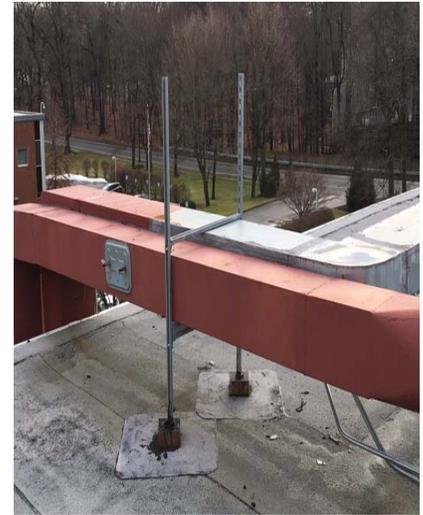
*Ductwork secured using brackets via pitch pockets*
