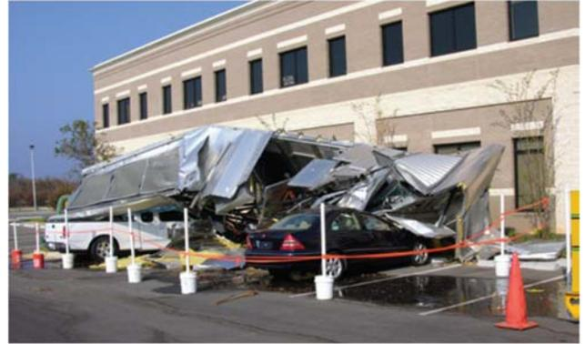
*Even larger, heavier equipment may be blown off the roof when securement is deficient.*
