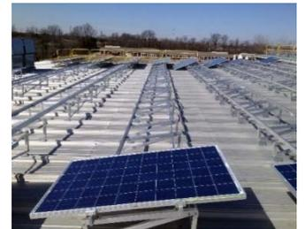
*While mechanically secured, this system lacks fasteners at every seam*
