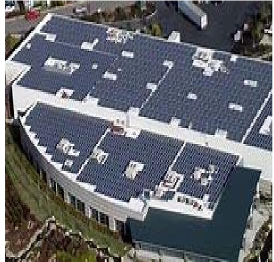
*Typical rooftop PV system with panels near the roof edges*
